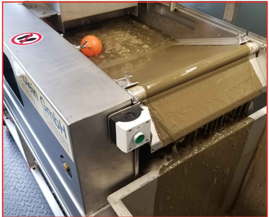
PFAS Sludge on Belt Filter
